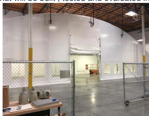
New 3,000+ sq ft WIAMan lab under construction at DTS
