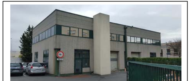
Located in Gennevilliers, the new DTS France Technical Center supports customers throughout Europe.
